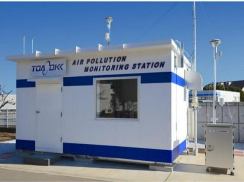
Air quality measurement station
