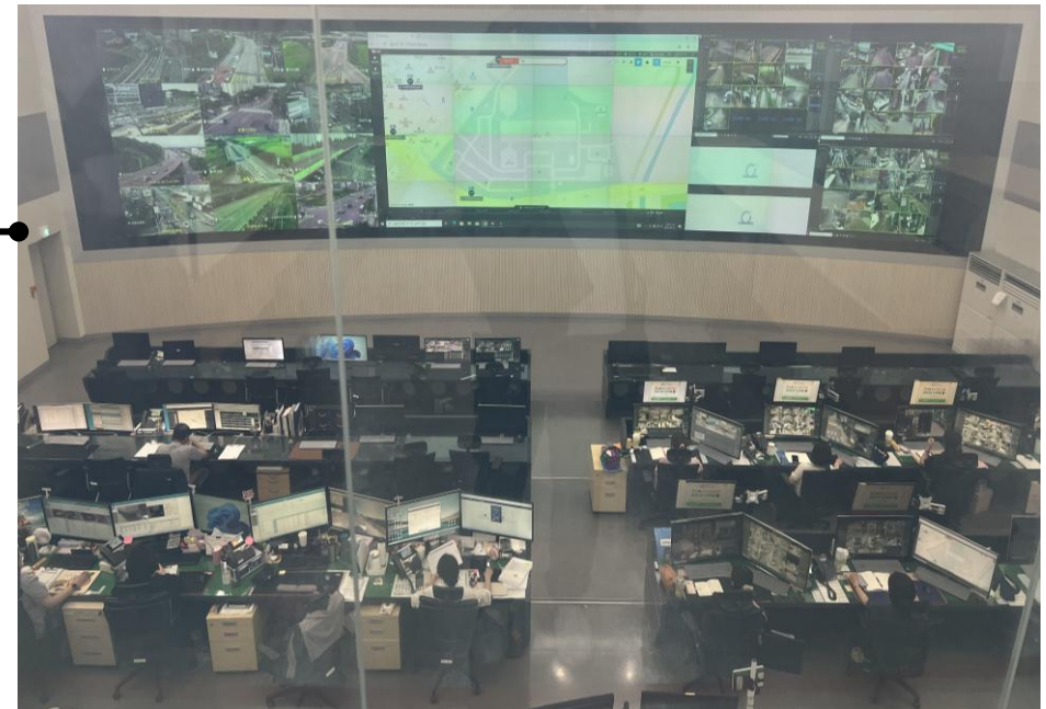
<Siheung Urban Integrated Information Center control room>
