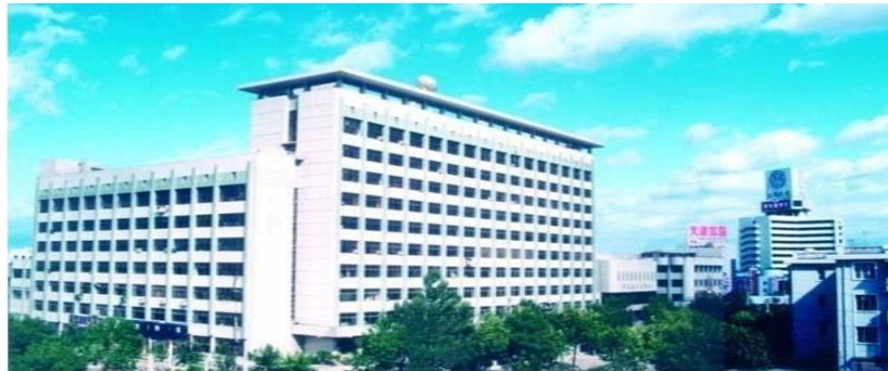
Office building in April 1989
