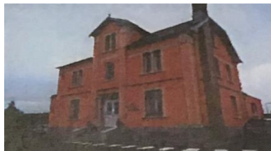
IME ADAPEI building
