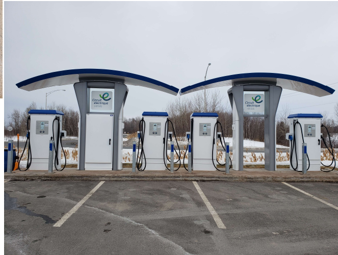
Superstation including four DCFC stations of 50kW each
