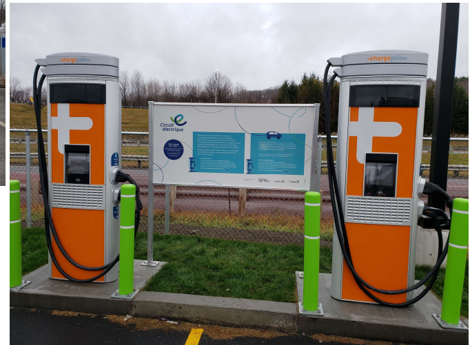
Superstation including four DCFC stations of 50kW each
