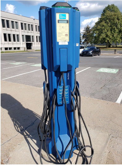
Level 2 public quadruple charging station providing power at 240V
