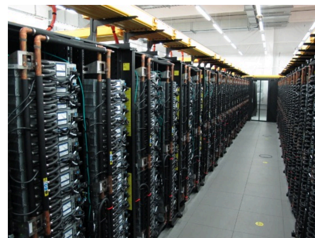
LRZ: Hot water cooling infrastructure (2012)
